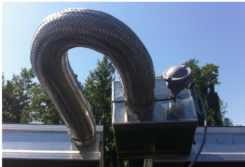
Figure 10: Temperature measurement at the mixed outlet of all rows of one collector array (left). Temperature measurement between collectors (right).
