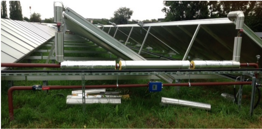
Figure 9: The volume flow sensors require settling sections upstream and downstream of the sensor.
